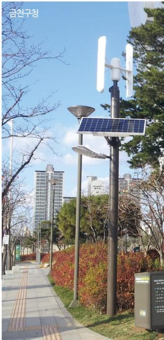
Generates power from hybrid system - wind(300W) & photovoltaic(200W)
